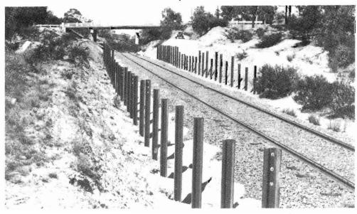
BUANGOR: Supports in place for sheeting a cutting as part of a stabilisation programme. Stabilisation is necessary in some areas to prevent tracks being covered by sand.
