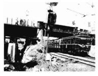
Reconstruction of the Hopkins Street (Footscray) bridge is well advanced. When the section on the left is completed and has services operating, the right-hand tracks will also be lowered to cater for additional head room.
