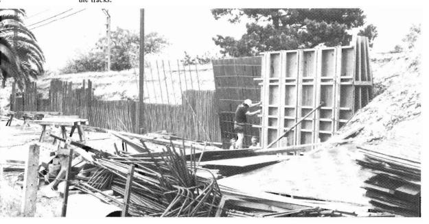
RETAINING WALL. A retaining wall is put into position between Ormond and Glenhuntly for the Mordialloc third track.
