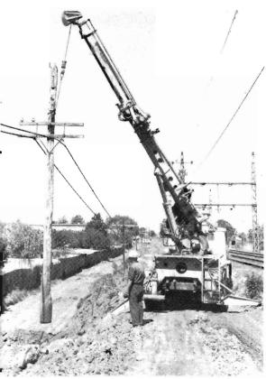
COMMUNICATIONS SHIFTOVER. A communications pole hangs suspended above the ground after being uprooted to make way for the third track to Mordialloc. The posts will be repositioned on the opposite side of the tracks.
