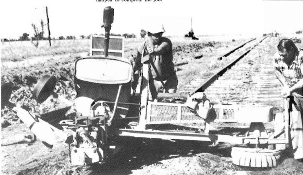
DENILIQUIN - MATHOURA: A mechanical adzing machine in use during track relaying operations. The machine is gui on one rail as it trims the other side of the sleepers before the second rail is spiked in place.
