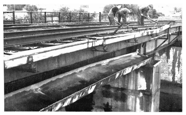
Victorian Railways staff make urgent track repairs after a truck has hit and damaged a bridge at Wantirna. Immediately above the displaced girder, signal cables have only just escaped damage.
