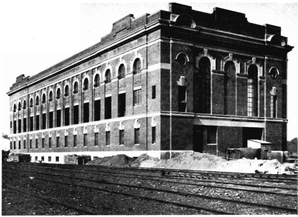
Demolition of the Jolimont sub-station is imminent. It was built between August 1914 and April 1915 to serve as a major electric power distribution point in the electrification scheme of the Melbourne suburban system, using 25 Hz power from Newport Power station. This fine building, which has been a landmark in Melbourne for 58 years, was one of a series of similar buildings built to house 20 000 V. switchgear and rotary converters supplying power to the overhead system.
