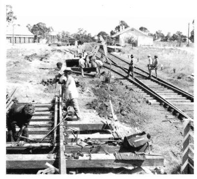
A "turnout" being built beside the main track at Bealiba, on the Mildura line, by the points and crossing gang under the control of Special Ganger Ken Snowden.
