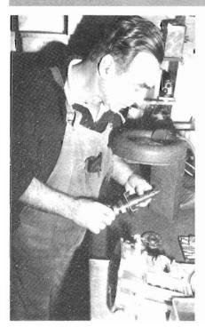
Plant fitter Carl Klissner examines a tractor part under an illuminated magnifier. He works on setting and adjusting fuel pumps most of the time.
