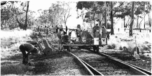
ANTWERP: Track relaying. The dog-spiking machine in the foreground is used to fix the rails in position.
