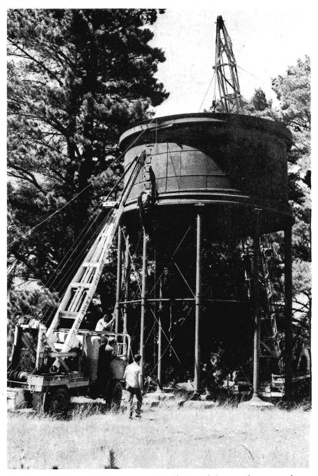
1874 WATER TANK REMOVED. Creswick's 104,558 litre capacity water tank, built 100 years ago and not used by the Railways since the 1940's, was dismantled last month. It was bought by Mr. L. R. Davies, of Ballarat, to be re-erected on a farm at Kooroocheang.
