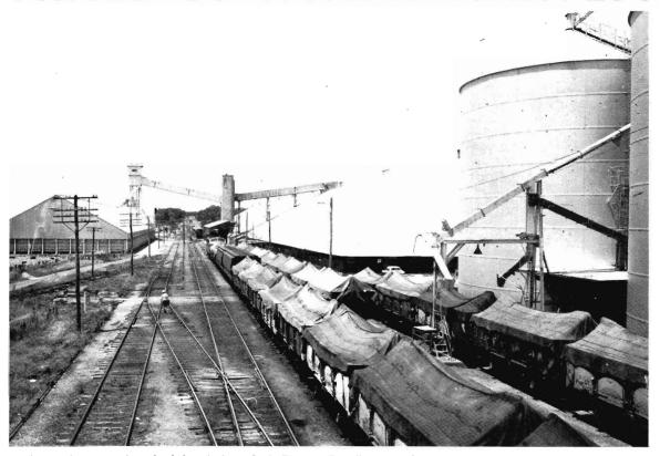
Wheat trains wait to be unloaded at the huge Grain Elevator Board's silos at Dunolly. The silos have an overall capacity to handle 323 700 tonnes of grain. Of this, the silo on the right can take 272 100 tonnes, the two local storage bins at front right 3 900 tonnes, and the silo on the left 47 700 tonnes. Dunolly receives grain to meet export and local requirements.
